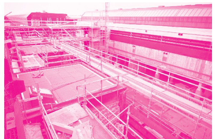
The five northernmost buildings in Farum Midtpunkt are completely renovated to remove PCBs. / © Enemærke & Petersen
